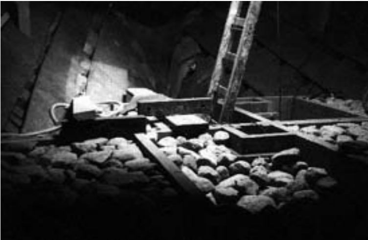
Abb. 20: The ballast before layering the floor
