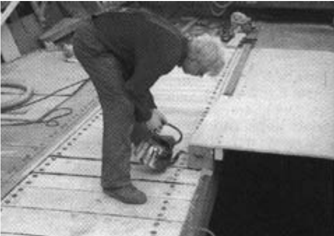
Abb. 12: The deck is sealed
